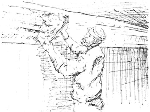
nario, modern clay-tile flue liners should be inserted in the chimney to refireproof it. A chimney sweep using a mirror attached to a string can assess the condition of an old flue, or tell you if a rebuilt flue needs cleaning.
