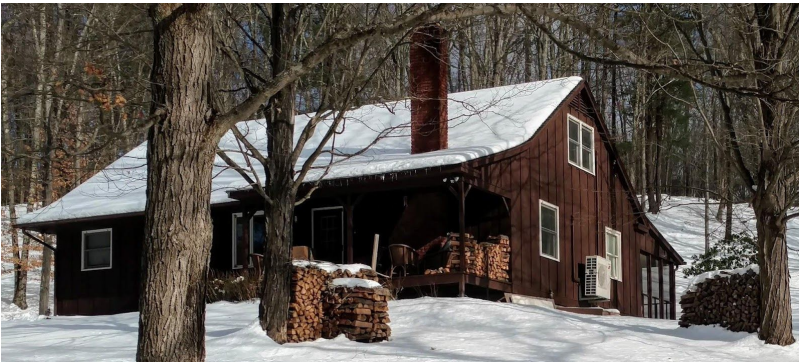
This Marbletown home demonstrates two forms of renewable heating: an air source heat pump and biomass heat from wood.
