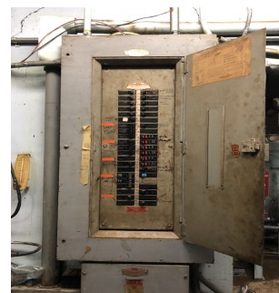
Old electrical panels and service that need to be replaced and updated to meet increased demand.
