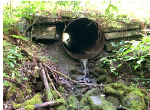
Figure 1 Can aquatic animals get through this culvert? Credit: Ben Ganon
