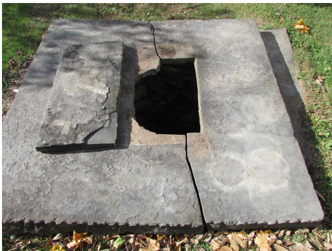
Below: Well with bluestone cover and inside stonework (pipes no longer functional).
